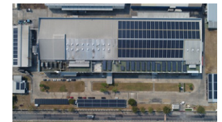
Solar panels installed at the NISSIN FOODS (Thailand), Nava Nakorn Plant
